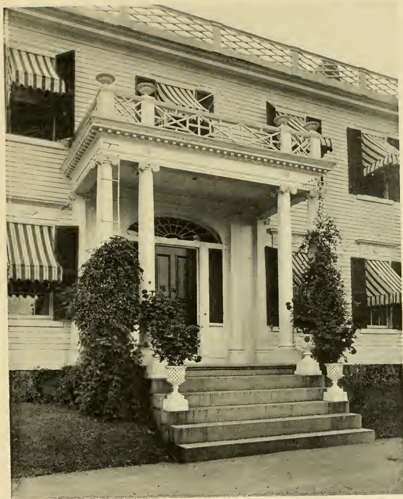
PLATE XXII. — Doorway, Rogers House.
